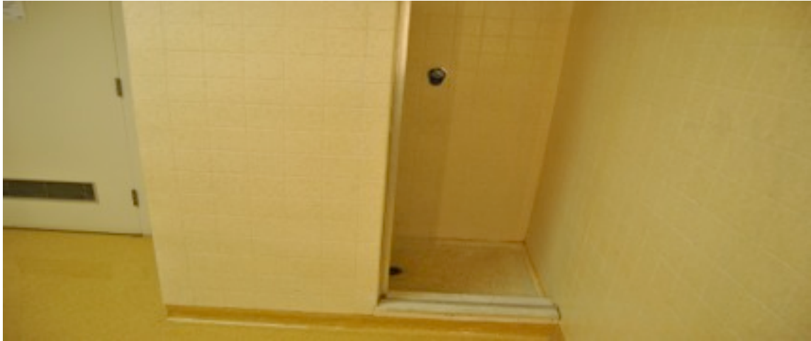
Sexton Library Building Complex Women's Locker Room
